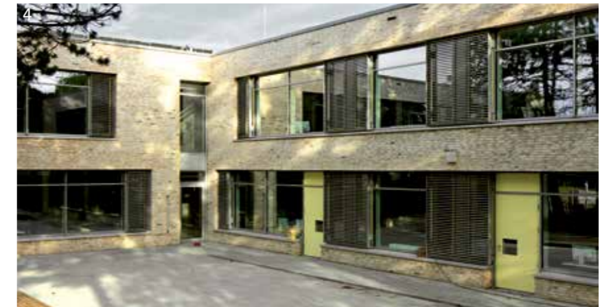
2 + 4 + 6. Extension of the Margarete-Steiff school in Möhringen (GER). Complete service package for 2.300 linear meters of timber-glass façade: planning, material supply, pre-fabrication, transport, and assembly of façade including fix and movable sun protection systems.
