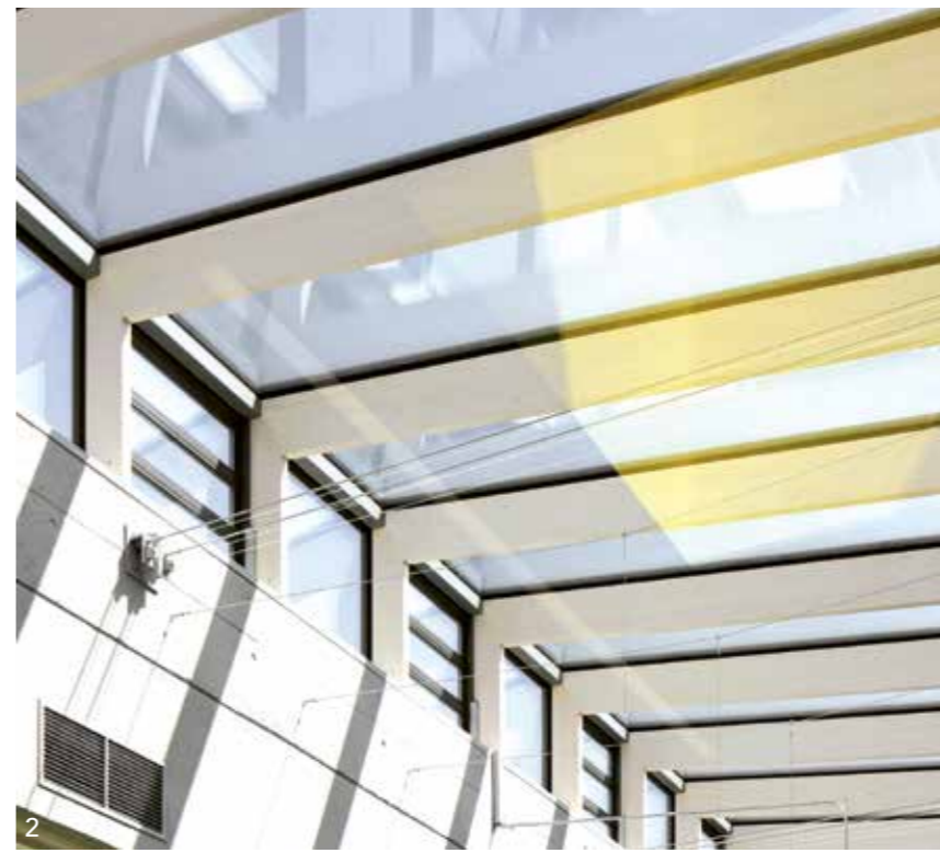
1 + 5 Extension of the secondary school complex Wiener Neustadt (AT). Two new building elements with 654 linear meters of timber-glass façade and roof glazing.
