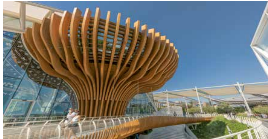
Oman Pavilion: Glued laminated timber: 275 m 3 Cross laminated timber: 60 m 3
