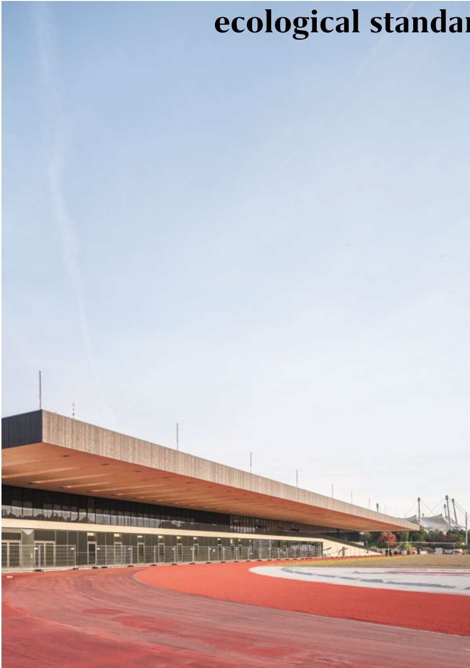
03 | TUM Campus in the Olympiapark The complex wooden roof structure cantilevers more than eighteen metres.
