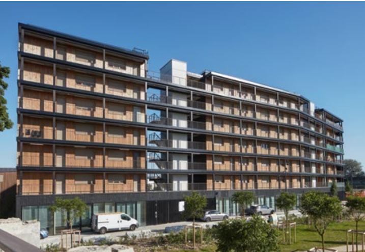
05 | ZAC Boissière Façade elements in timber frame construction, pergolas and balconies made as timber-concrete construction.
